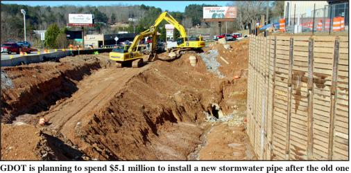
burst in a rainstorm last August, contributing to a massive sinkhole at Murphy Highway and
